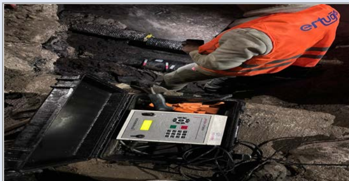
ANADOLU YAKASI KÜÇÜKBAKKALKÖY HİDRANT ONARIM İŞİ
