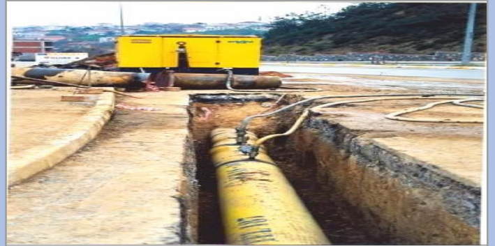
İSTANBUL & BOĞAZİÇİ (170) DOĞALGAZ BORU HATTI PROJESİ
